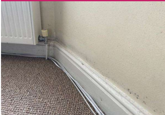
21-11-2022 12:34 / Walls Ceilings / Poz7meqn5
