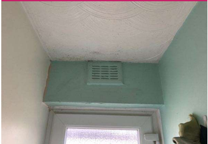
21-11-2022 12:38 / Stairs And Landing Photo / Hajllibe9
