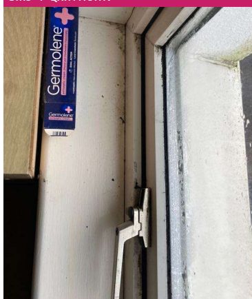
21-11-2022 12:41 / Bedroom Windows Sills / Qkif7homv
