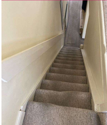
21-11-2022 12:39 / Stairs And Landing Photo / Rtiakkt8j
