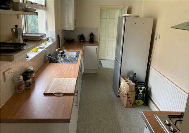
21-11-2022 12:36 / Kitchen Condition / 050cply
